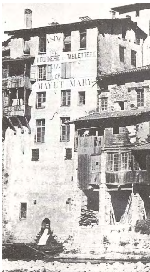
Figure 24 L'usine Mary Mayet
